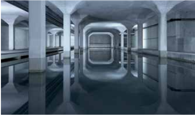
Cover: Hardhof Lengg © Luca Zanier
